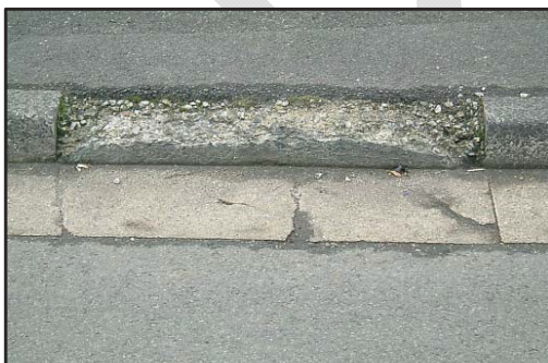
Kerb vertical projection, damaged or missing (EVPJ, DAMG, MISS)
